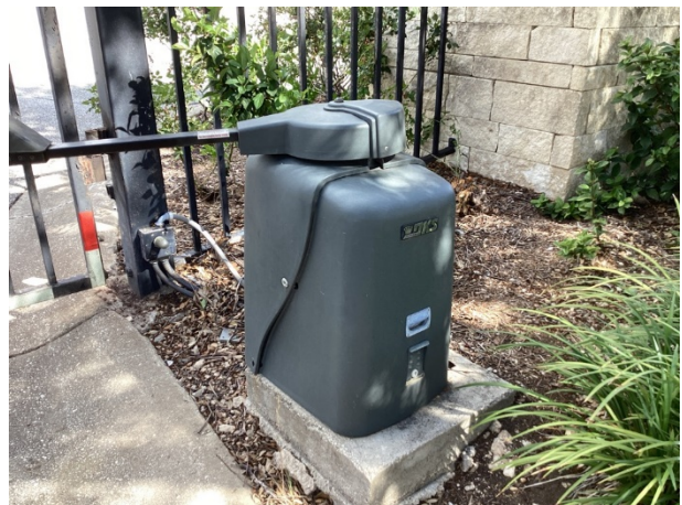
Typical gate operator at the property
