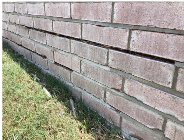
Wall exposed support wire
