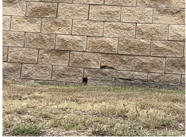
Wall brick spalls at the Peak
