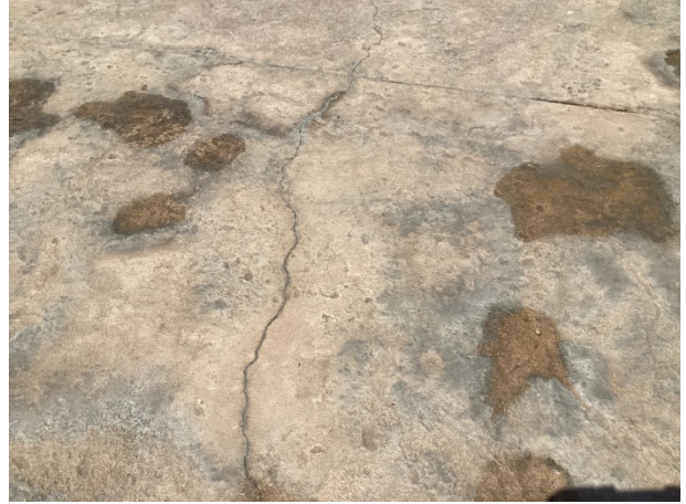
Concrete cracks
