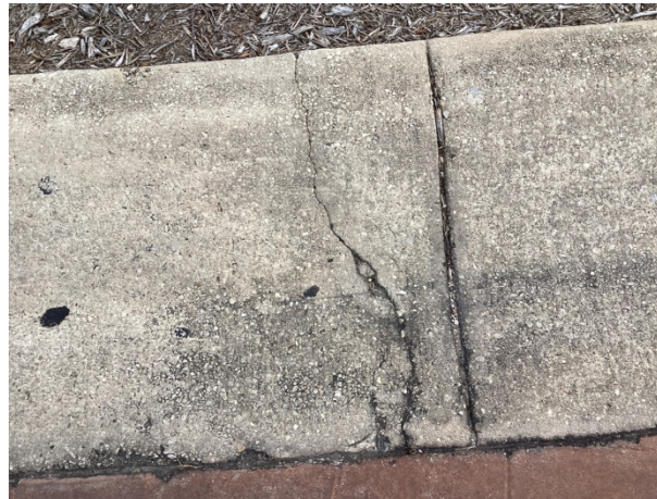
Concrete cracks at the Peak
