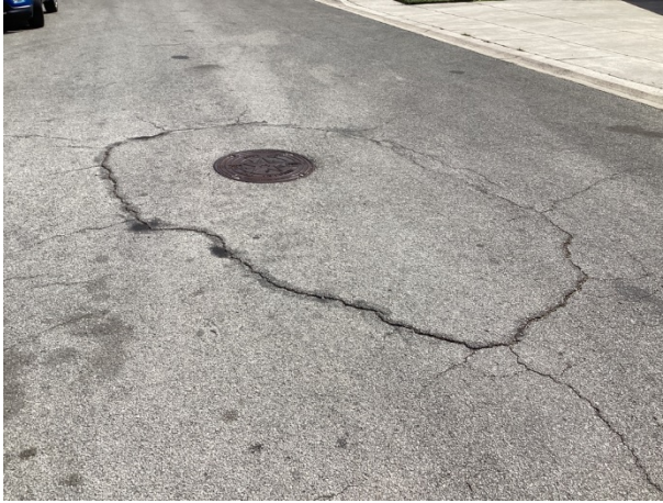
Pavement cracks at the Heights
