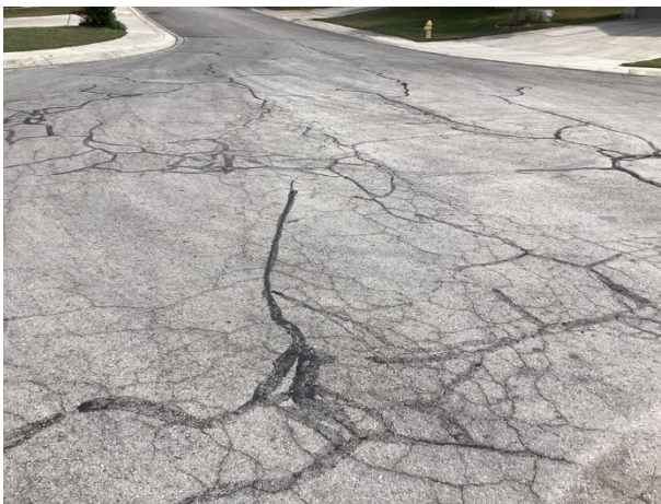
Alligator cracks and previous repairs at the Reserve
