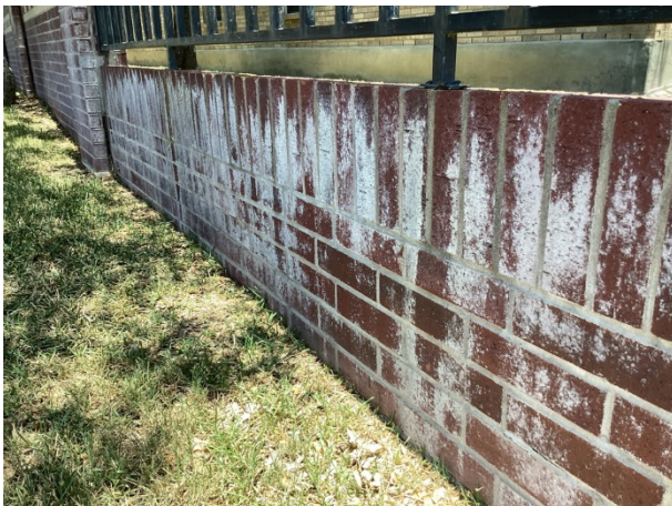
Wall efflorescence
