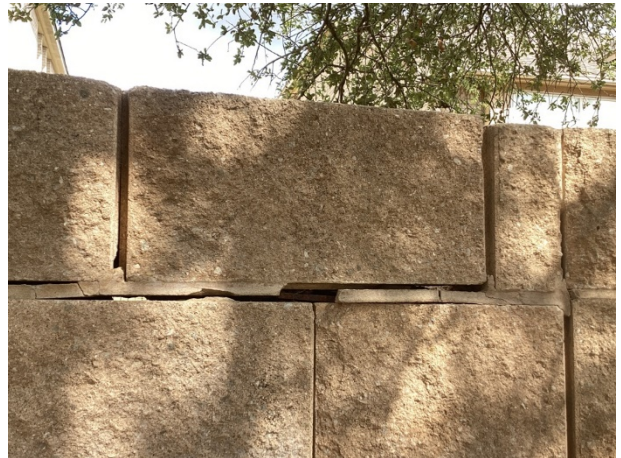
Wall mortar deterioration and exposed reinforcing steel at the Heights
