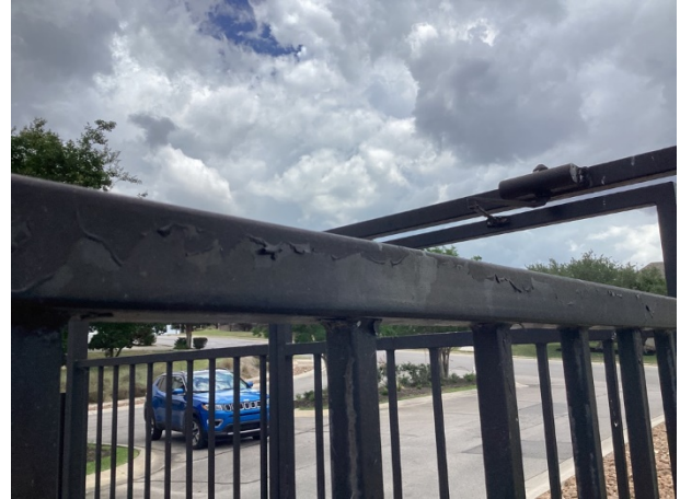
Fence finish deterioration at the Peak
