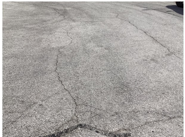
Pavement cracks at the Preserve
