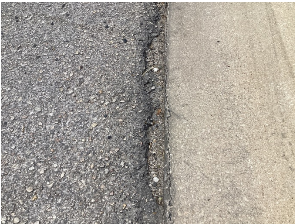
Edge deterioration at the Peak
