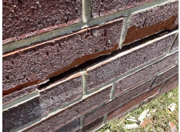
Wall exposed support wire
