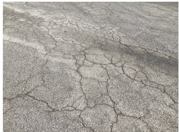
Alligator cracks at the Heights
