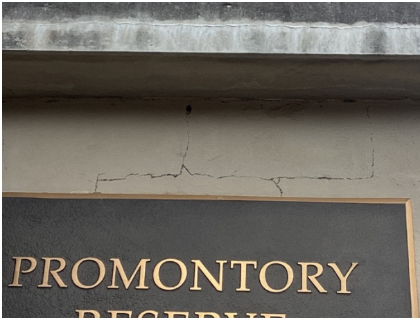
Wall stucco cracks at the Reserve
