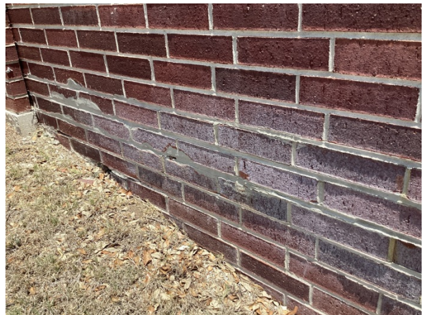
Wall efflorescence and previous repairs
