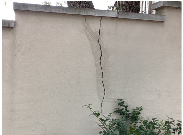
Wall stucco cracks at the Peak
