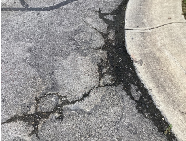
Pavement cracks and edge deterioration at the Peak
