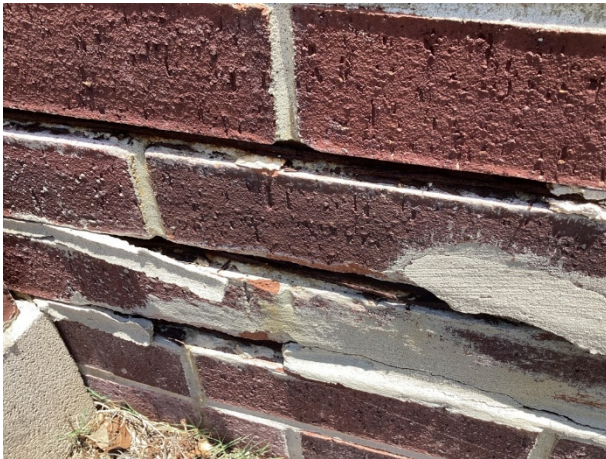
Wall exposed support wire
