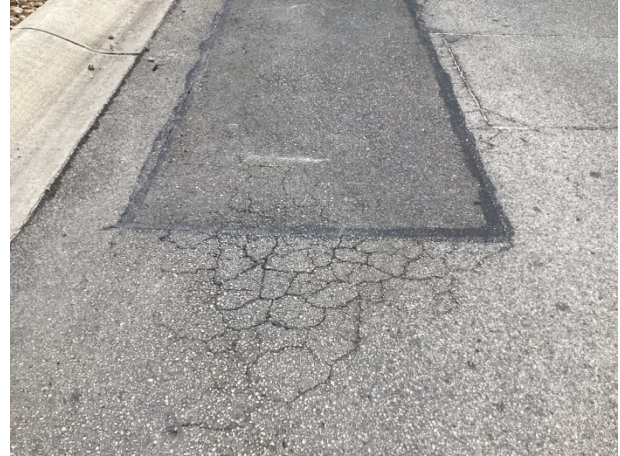
Alligator cracks at previously patched section at the Peak
