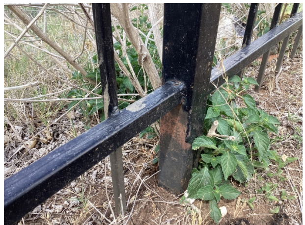
Fence finish deterioration and rust at the Reserve
