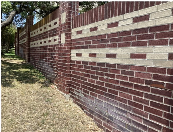
Panelized masonry perimeter wall along Knights Crossings
