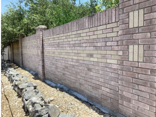
Panelized masonry perimeter wall along Bear Ridge
