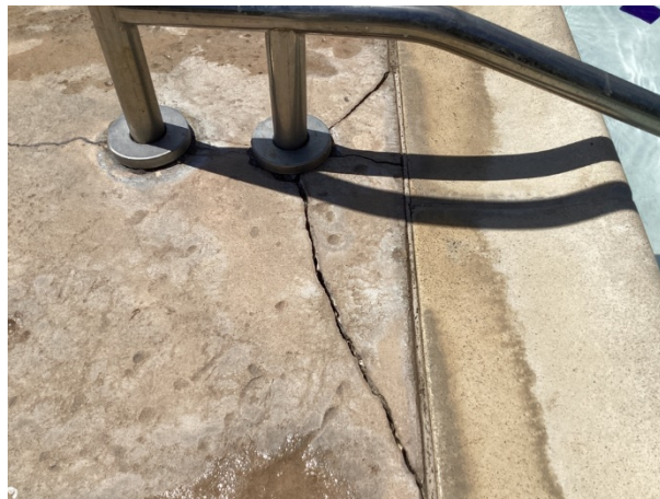
Concrete cracks
