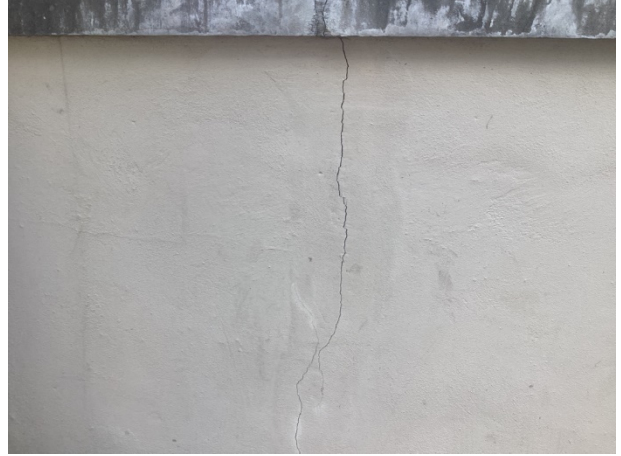
Wall stucco cracks
