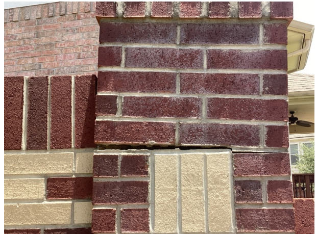
Damaged column
