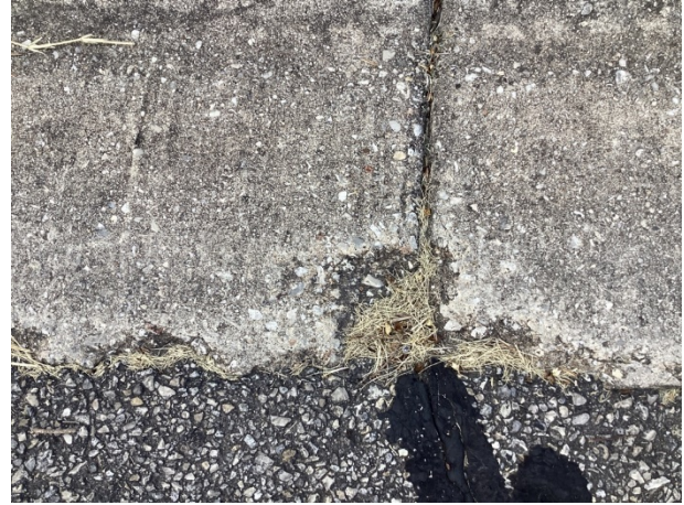
Concrete spalls at the Reserve
