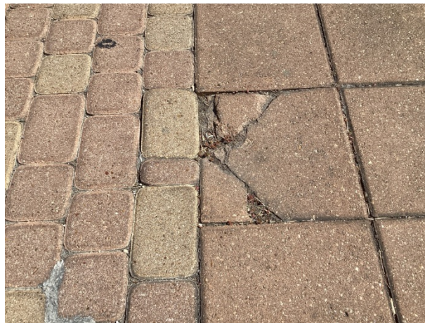
Damaged pavers at the Reserve
