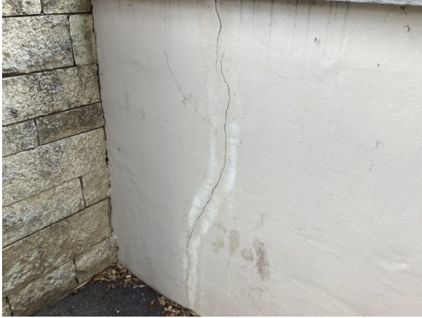
Wall stucco cracks
