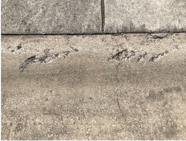
Concrete spalls and cracks
