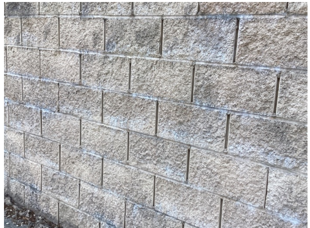
Wall efflorescence
