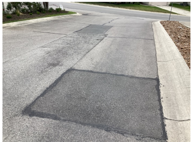
Previous repairs and alligator cracks at the Peak
