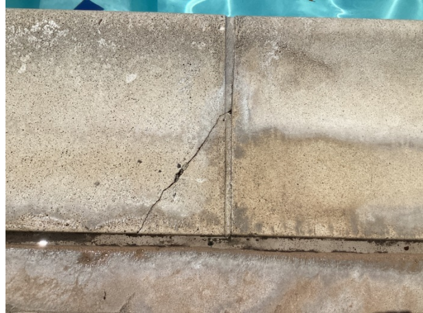
Pool coping cracks
