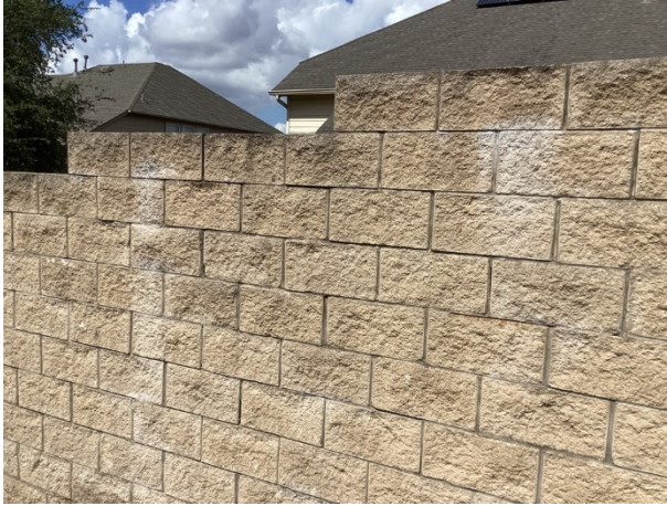
Wall efflorescence
