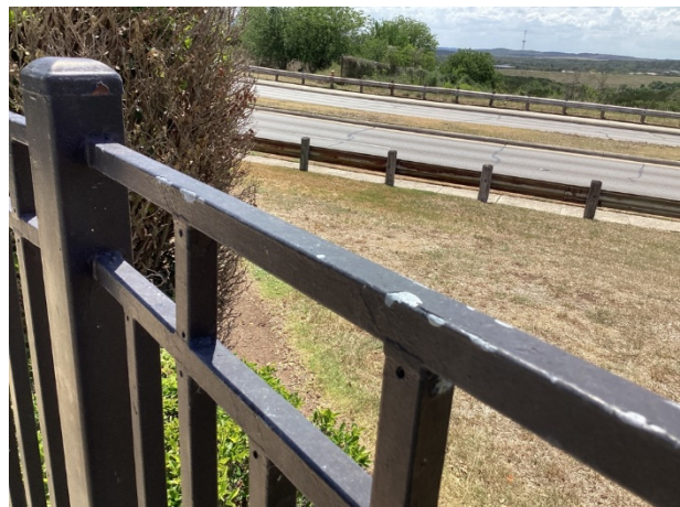
Fence finish deterioration
