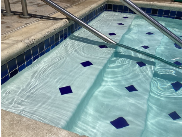
Pool plaster finish with tile perimeter
