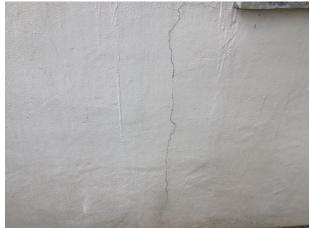
Wall stucco cracks
