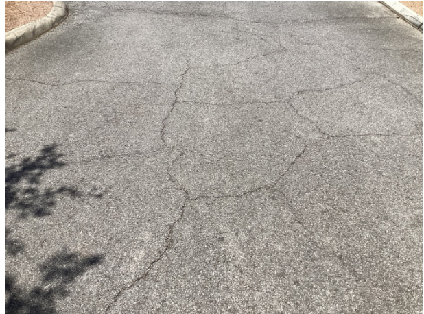
Pavement cracks at pool parking area
