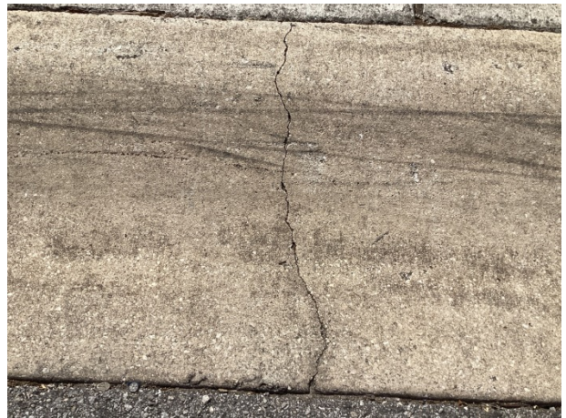
Concrete cracks
