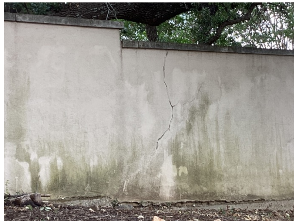
Wall stucco cracks at organic growth at the Peak
