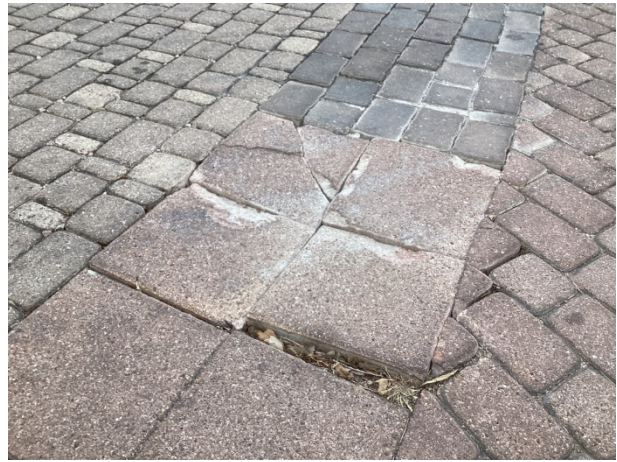
Damaged pavers at the Heights
